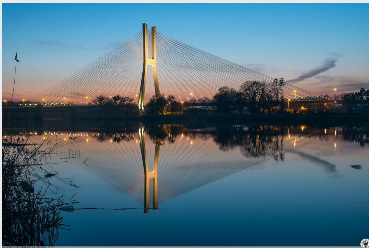
Rędzki Bridge. The bridge is the longest cable-stayed bridge with one pylon in Poland.
